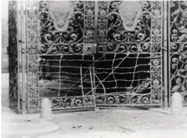
Figure 2.4. Damaged gates at Newnham College. With permission from Newnham College, Cambridge.
