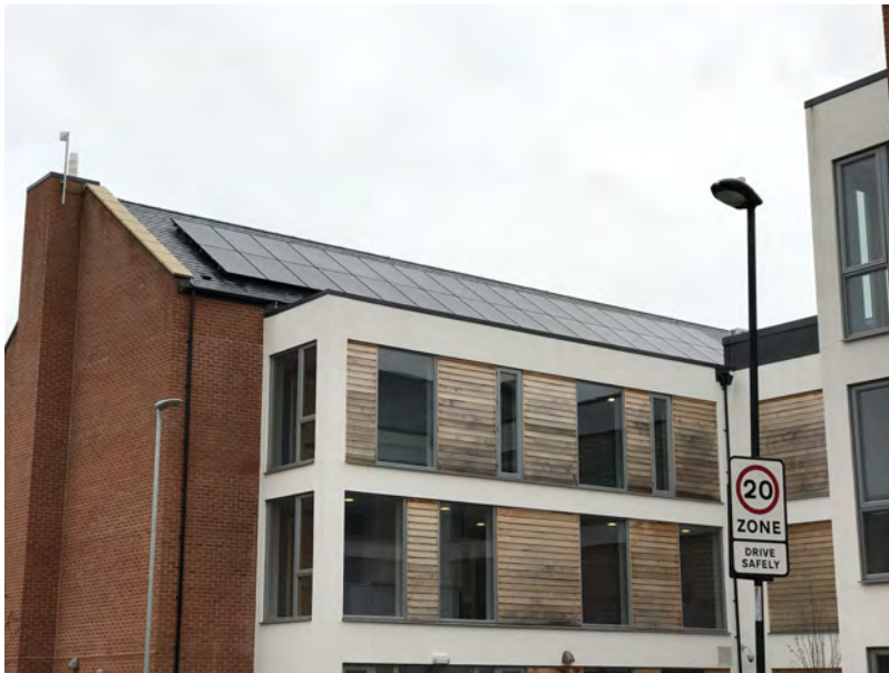
Figure 7.4. Solar panels, double glazing, and LED energy saving light at the retirement accommodation Whinstone Lodge, in Whitley Bay in the UK. (© Dr Alex Hope. Reproduced with permission.)
