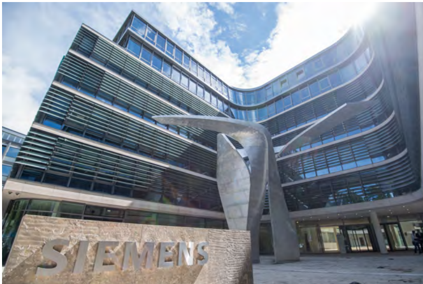
Figure 7.7. The Siemens HQ in Munich, Germany. It consumes 90% less electricity and 75% less water than its predecessor, and has a platinum LEED certification, which is the highest level possible. Its sustainability features include solar cells on the roof that generate around a third of the required electricity, a system that collects rainwater for flushing toilets and watering the grounds, triple glazing angled such that the amount of natural light entering the building from the inner courtyards is maximised and artificial lighting use is therefore reduced, and the use of regionally-quarried natural stone tiles for parts of the exterior and flooring. (Courtesy of Siemens. www.siemens.com/press .)
