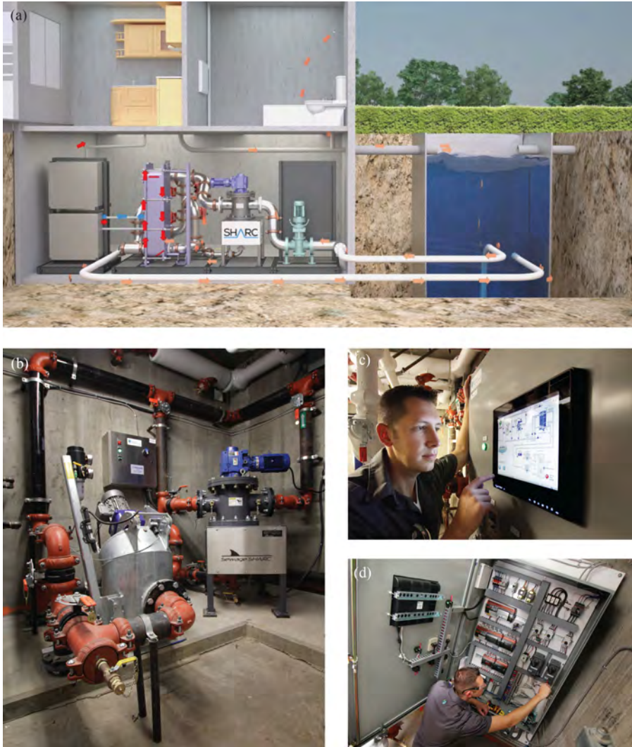
Figure 7.5. The SHARC sewage heat recovery system. (a) Diagram showing the fluid flow through a SHARC system installed in a house. (b)–(d) The SHARC system in the Sail Condominium Project at the University of British Columbia in Canada. This installation is producing hot water for the building as well as heating it via an under-floor heating system. It is generating 220 000 BTU every hour, and reducing carbon emissions by 100 tonnes a year. (Courtesy of IWS. Reproduced with permission.)
