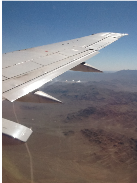
Figure 6.12. Ivanpah solar thermal towers in southern California seen from an airplane. Each of the bright spots is one tower surrounded by 173 500 mirrors which reflect the Sun's energy onto the tower. (Photograph taken by the author.)
